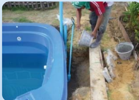
06. Begin filling with water and back filling
