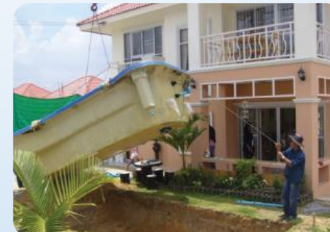
04. The Pool is lowered into the hole
