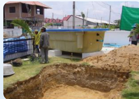
03. Hole Surface Preparation and Sand Bed
