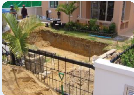
02. Ground Preparation and Excavation
