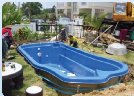
05. Filtration, Plumbing and Light installation
