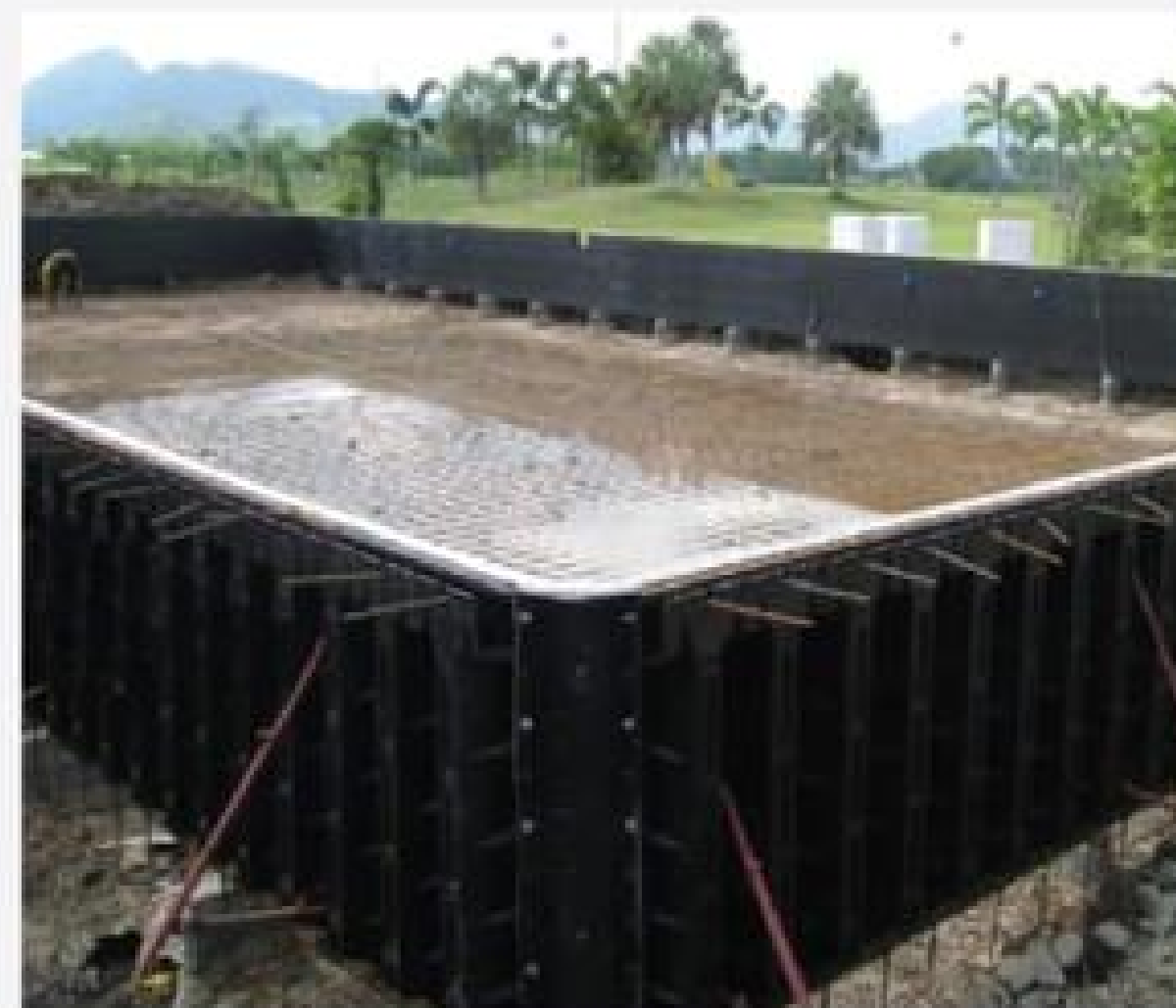
Concrete Structure with Injection Panel 10-30 days
