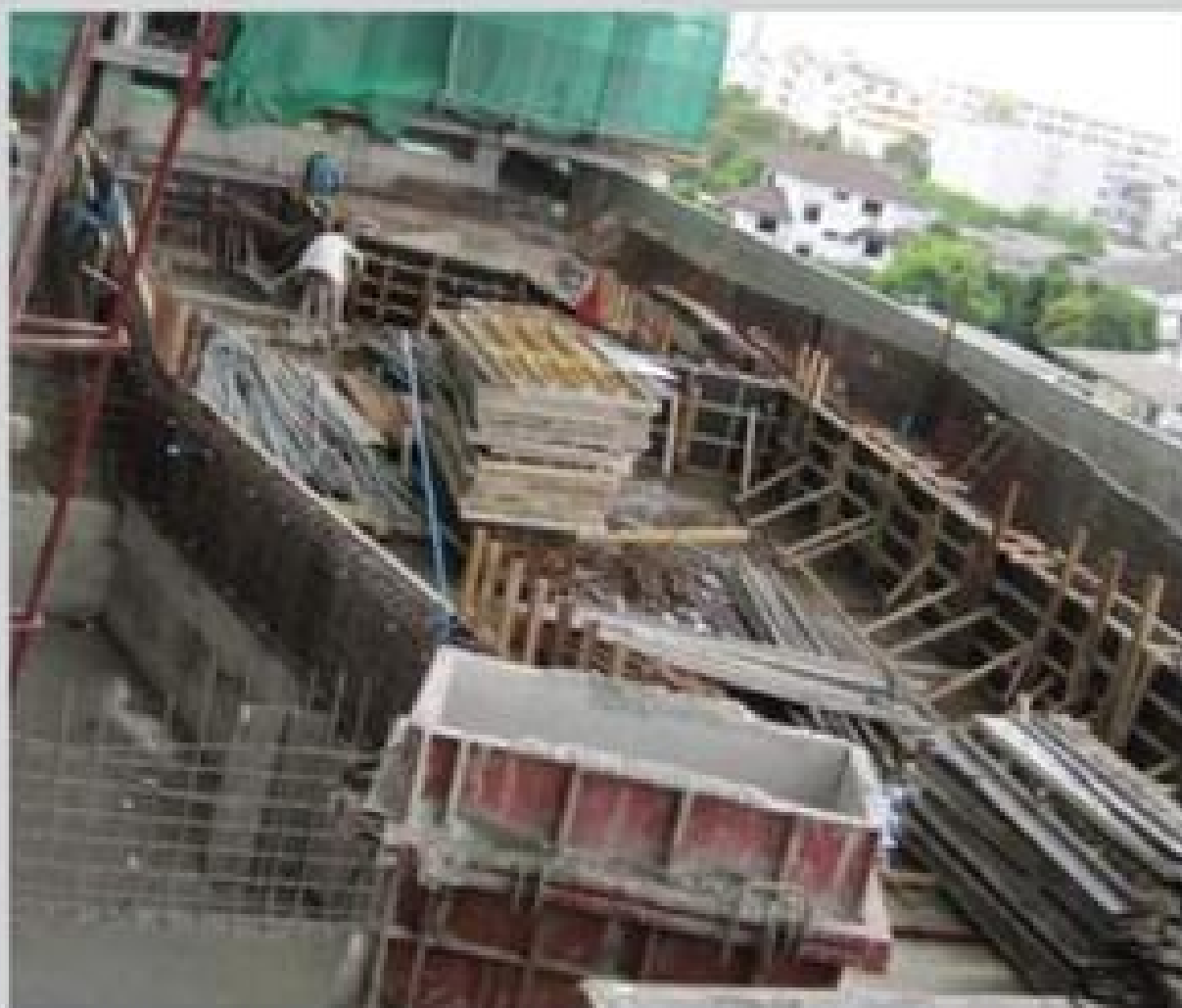
Concrete Structure from Wooden Framework 90-120 days
