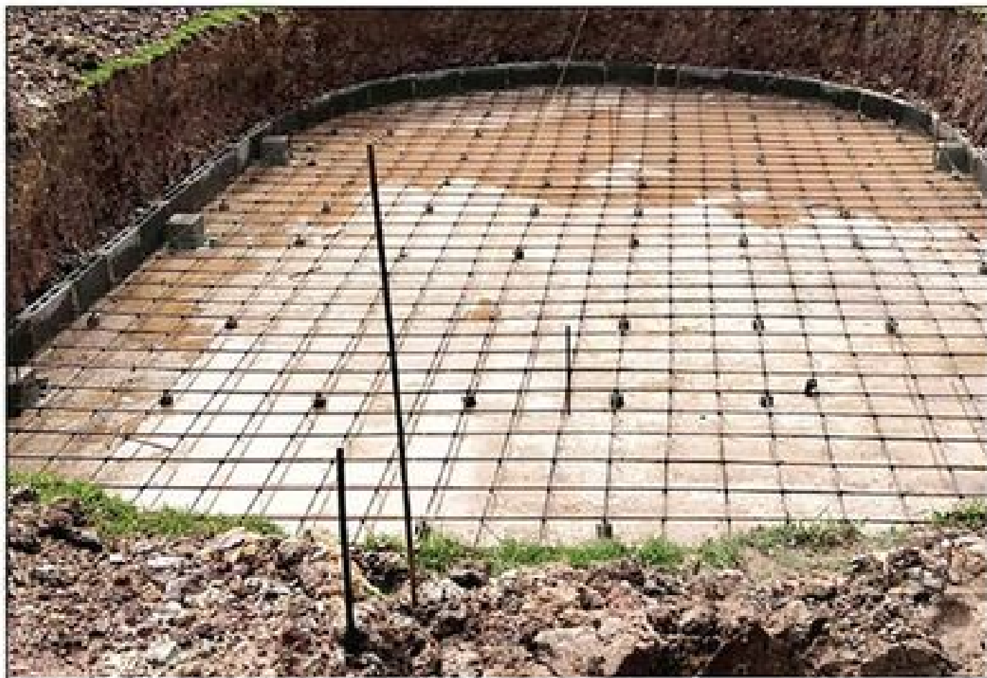
Pool Base Preparation Lay the floor reinforcement (RB9 wire mesh at 20 cm spacing) to help distribute the load, reduce cracking and increase the floor's strength.
