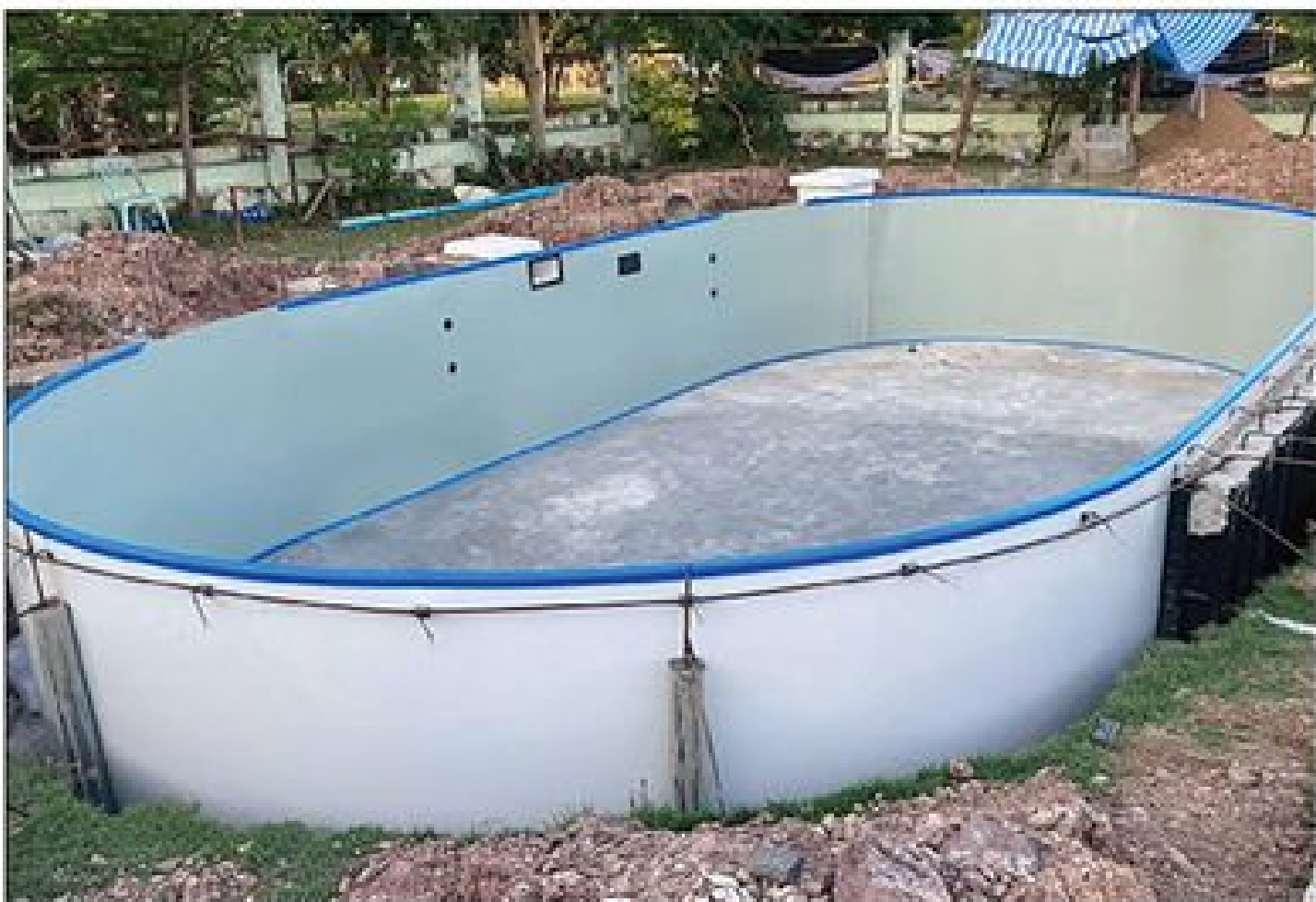
Install the iSteel Pool Walls Check and adjust the wall alignment so the pool sits perfectly level, ready for the interior finishing stage.
