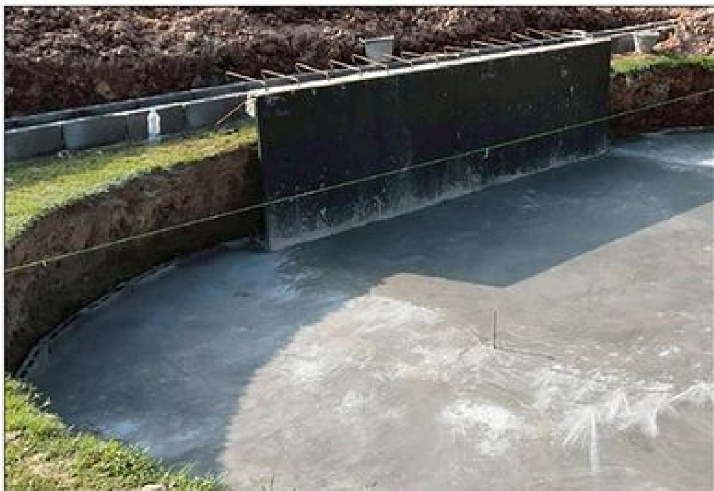
Pour Concrete for Walls and Base Pour concrete for the floor and walls to lock the entire structure in place. Trowel-polish the pool floor to a smooth, even finish.
