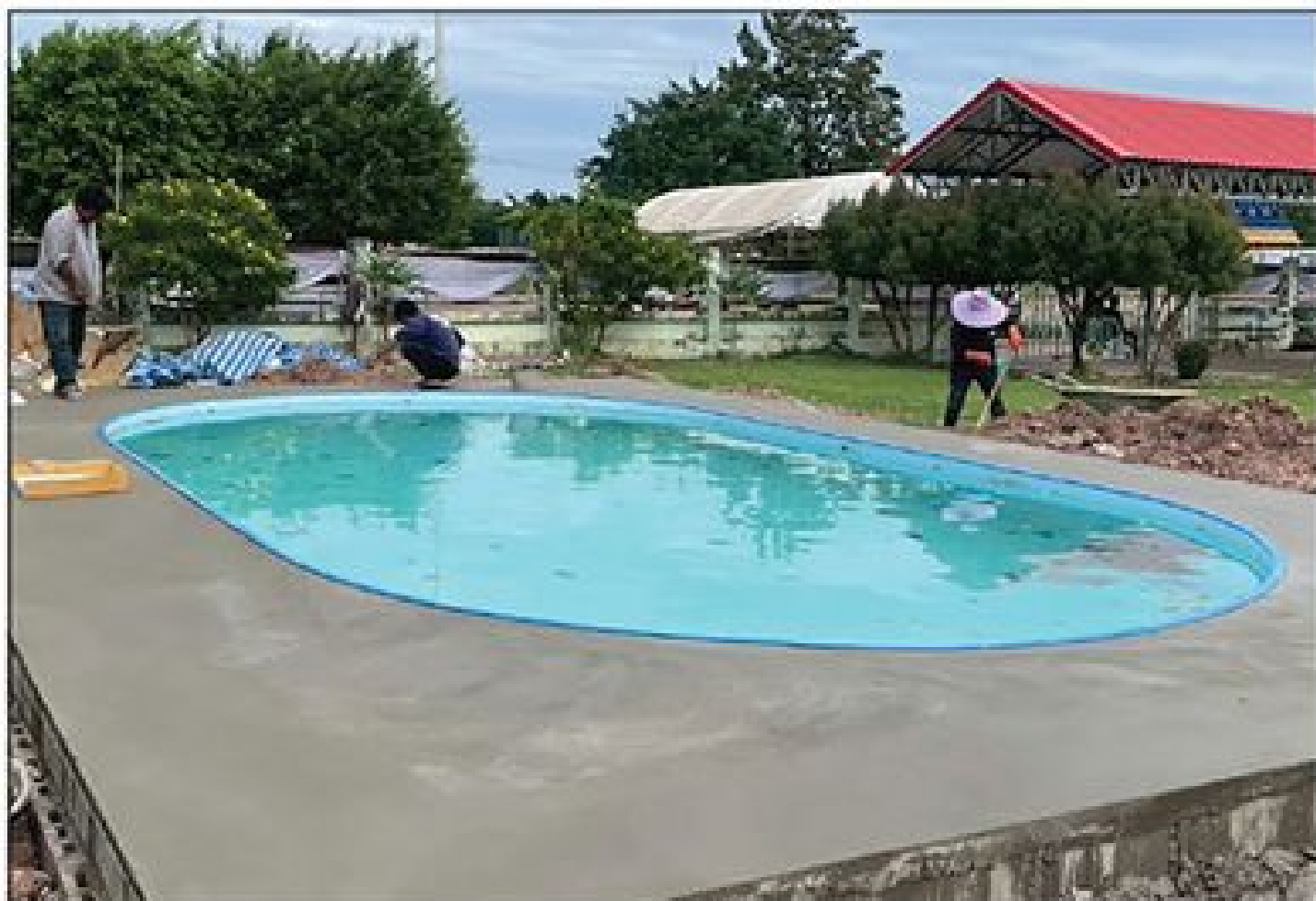
Install Lighting, Plumbing and Surrounding Finishes Fill the pool with water and squeeze out any air bubbles under the liner so it sits perfectly smooth and wrinkle-free. Run the underwater lighting and plumbing, and finish the deck around the pool.
