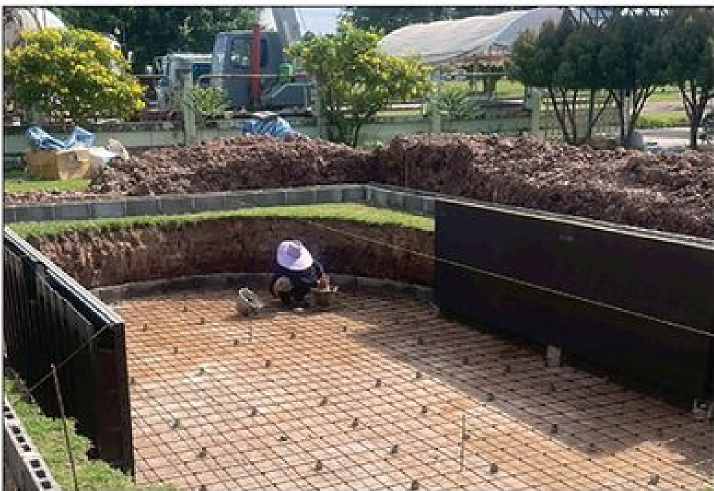
Install the iPanel Smart Wall Structure Install the iPanel structure to reinforce the sides of the iSteel pool.
