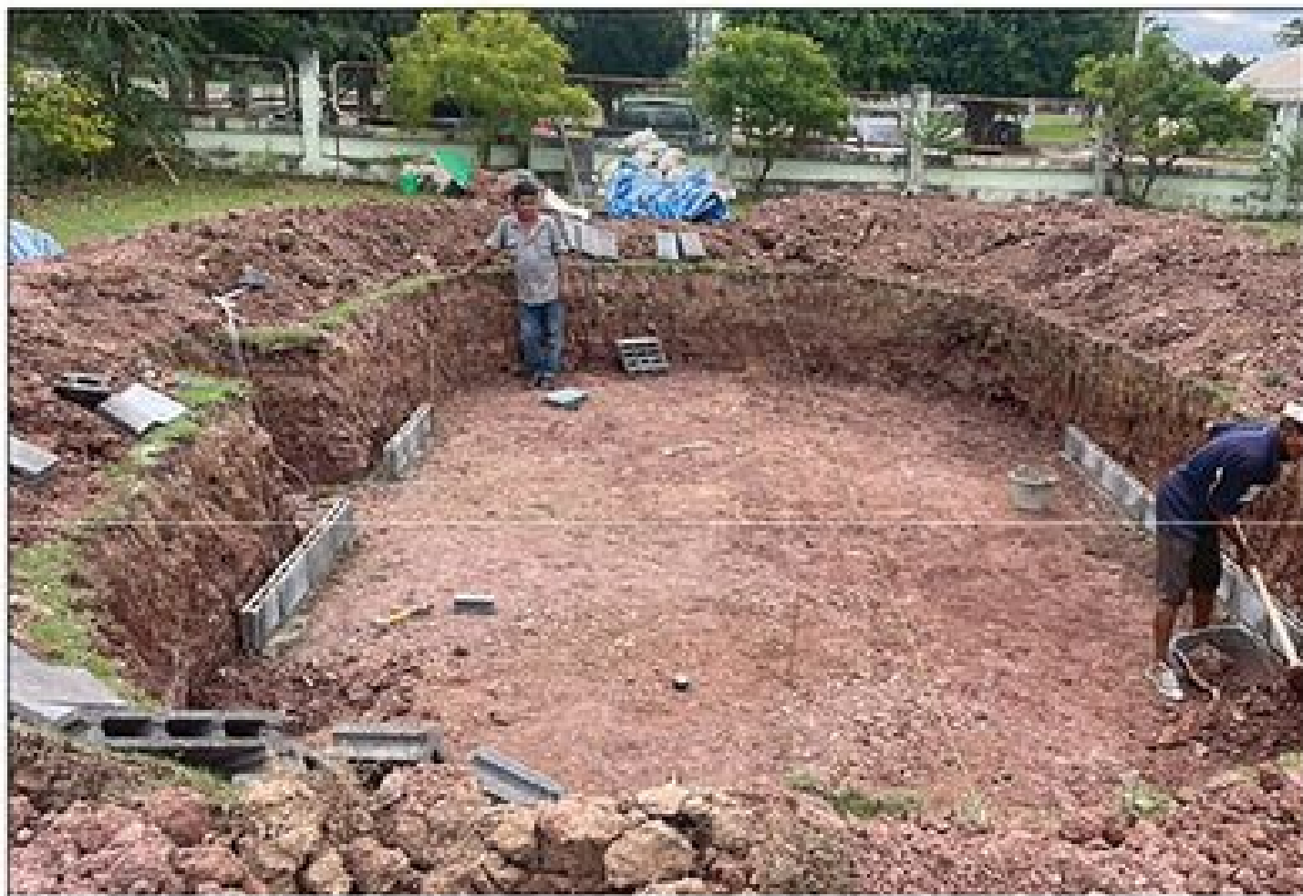
Excavation & Ground Leveling Excavate the pool pit to the specified dimensions and bring the floor down to 1.4 m below the reference ground level. Compact the soil evenly and firmly across the entire footprint, ready for construction.
