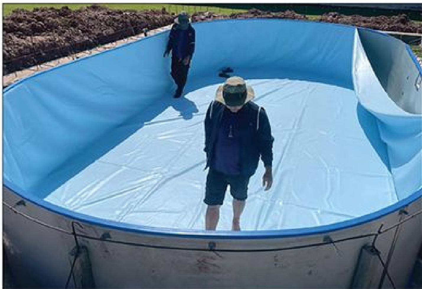
Install the Prefabricated PVC Liner Install the prefabricated PVC liner, smoothing it tight against the floor and walls so there are no creases or wrinkles.
