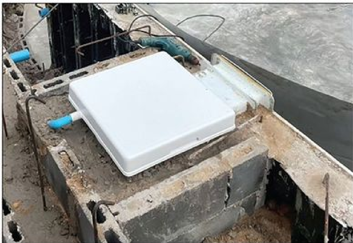
Install the Filtration System and Pool Equipment Install the filter unit and pump room, plus the plumbing and electrical systems.
