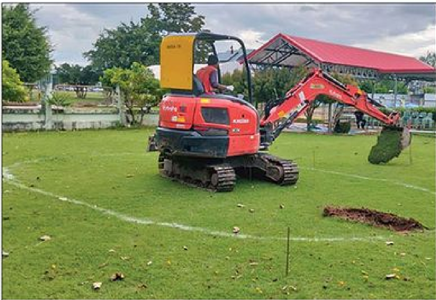
Layout & Pool Positioning The team arrives on site, takes measurements, and sets the pool's position, depth and orientation to match the design and the available area.
